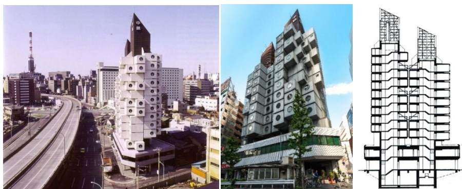
Slika 8. Nakagin hotel kapsula: a) i b) spoljašnji izgled c) presek. Izvor: http://www.noobz.ro/2013/10/01/capsule-tower-un-hotel-unic-in-lume-made-in-japan/
